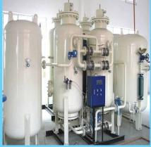
PSA type nitrogen generators are utilized extensively in food and beverage packaging, electronics manufacturing, chemical industries, medical facilities
